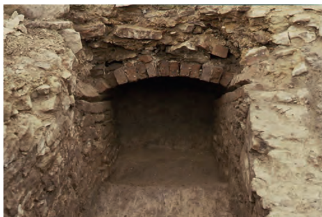
Fig. I/15: Chrudim, Filištinská St., cesspit XVIII. Drainage of sewage through the town wall with a brick arch. 16 th century.
